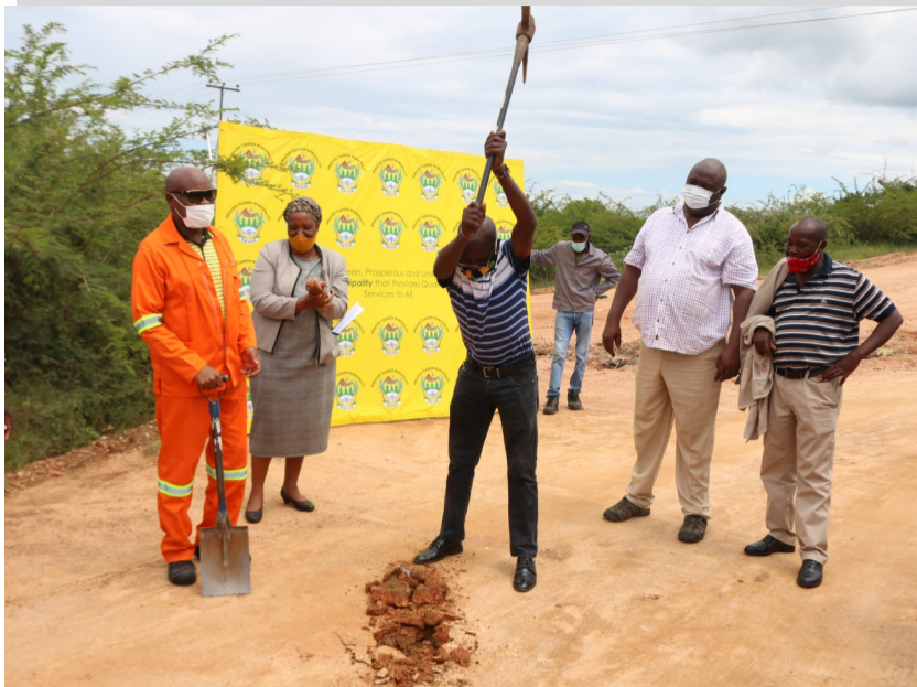
Mayor Maripe Mangena, Cllr. Sophy Raganya (Chairperson: Infrastructure Portfolio Committee), Cllr. Edward Ngobeni (Ward 13), Cllr. Edney Ntimbani (Head of Infrastructure), and Headman Xiake (Caswell Baloyi) during sod-turning ceremony at Jamba Bridge 8 February 2021
